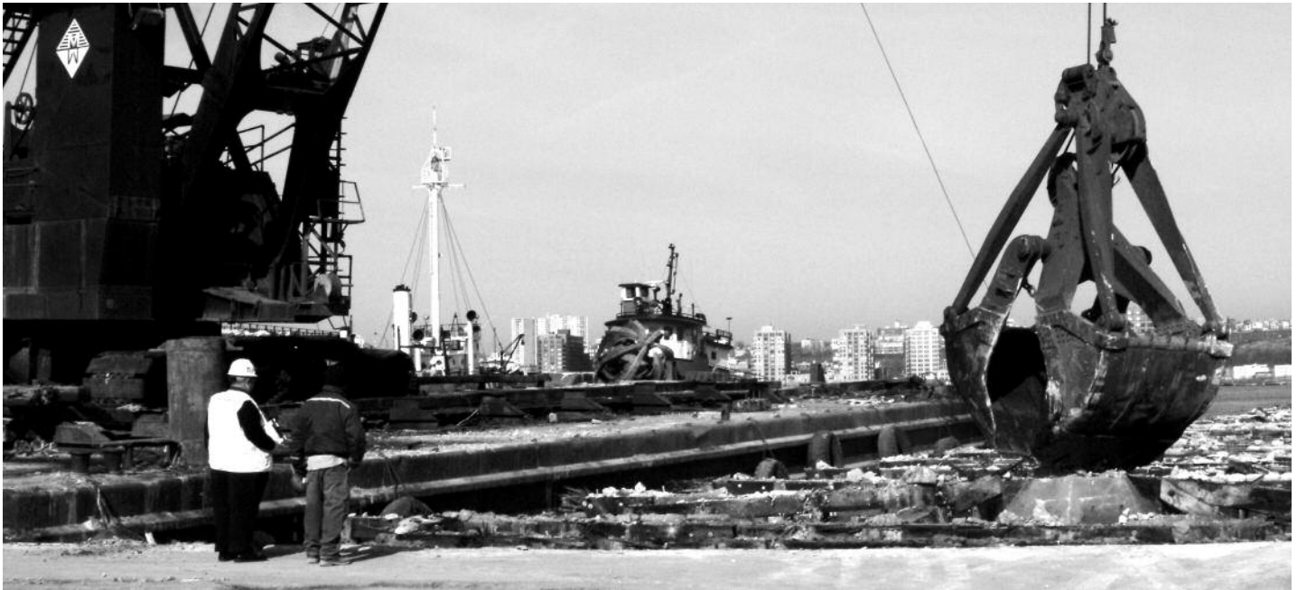
Pier 64's deck being removed, April 12, 2006.
