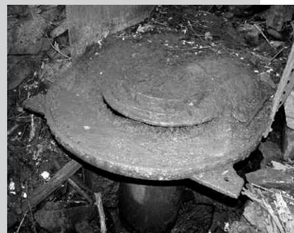
*RIGHT: With the sheet iron stripped away, the base for the second turbine is visible. One of the exit pipes leading to the tailrace is shown in the bottom center.*
