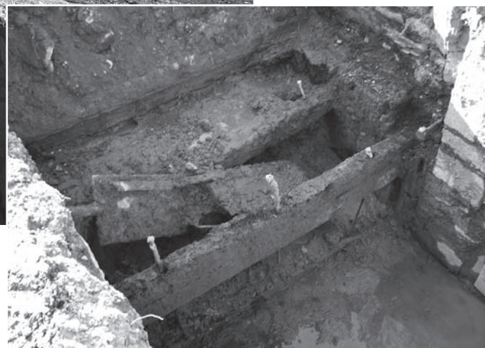
At the upper end of the lock, the wooden platform that supported wicket gates was found in tact, preserved in the wet soil at the bottom of the lock. In the picture below one of the wicket's iron shutter valves can be seen knocked askew by falling stones.
