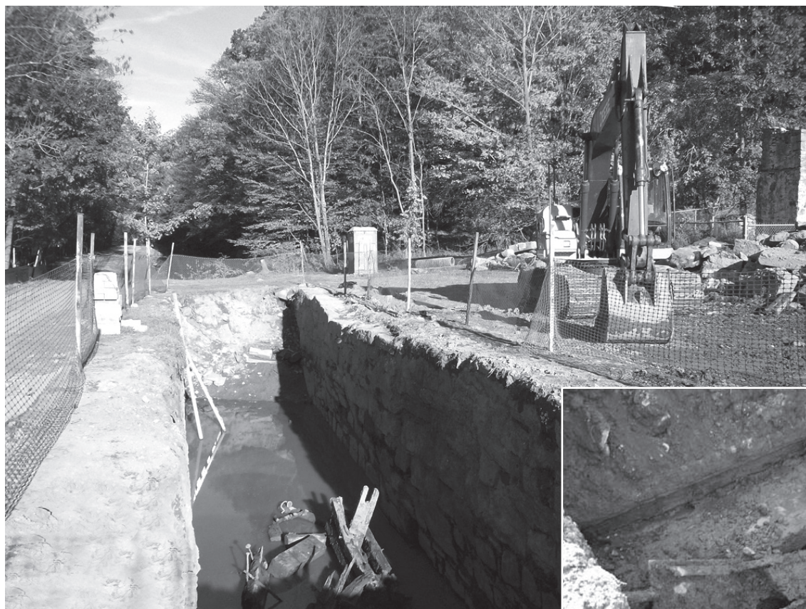
When Morris Canal Lock 2 East was abandoned in the 1920s, the cap stone that formed the top edge of stonework were pushed into the lock and the chamber filled with earth. This fall workers started removing the dirt fill in preparation for rebuilding the lock.
