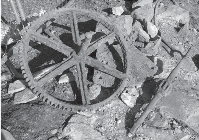
These gears are part of the rack and pinion the enabled the lock tender to crank both lower lock gates open and closed at the same time.
